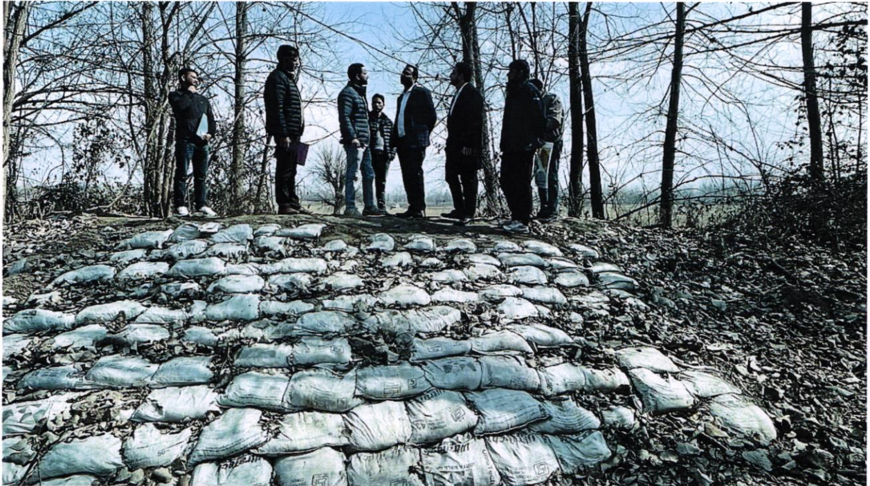
Photo 1. Embankment repaired by the Irrigation and Flood control department.
