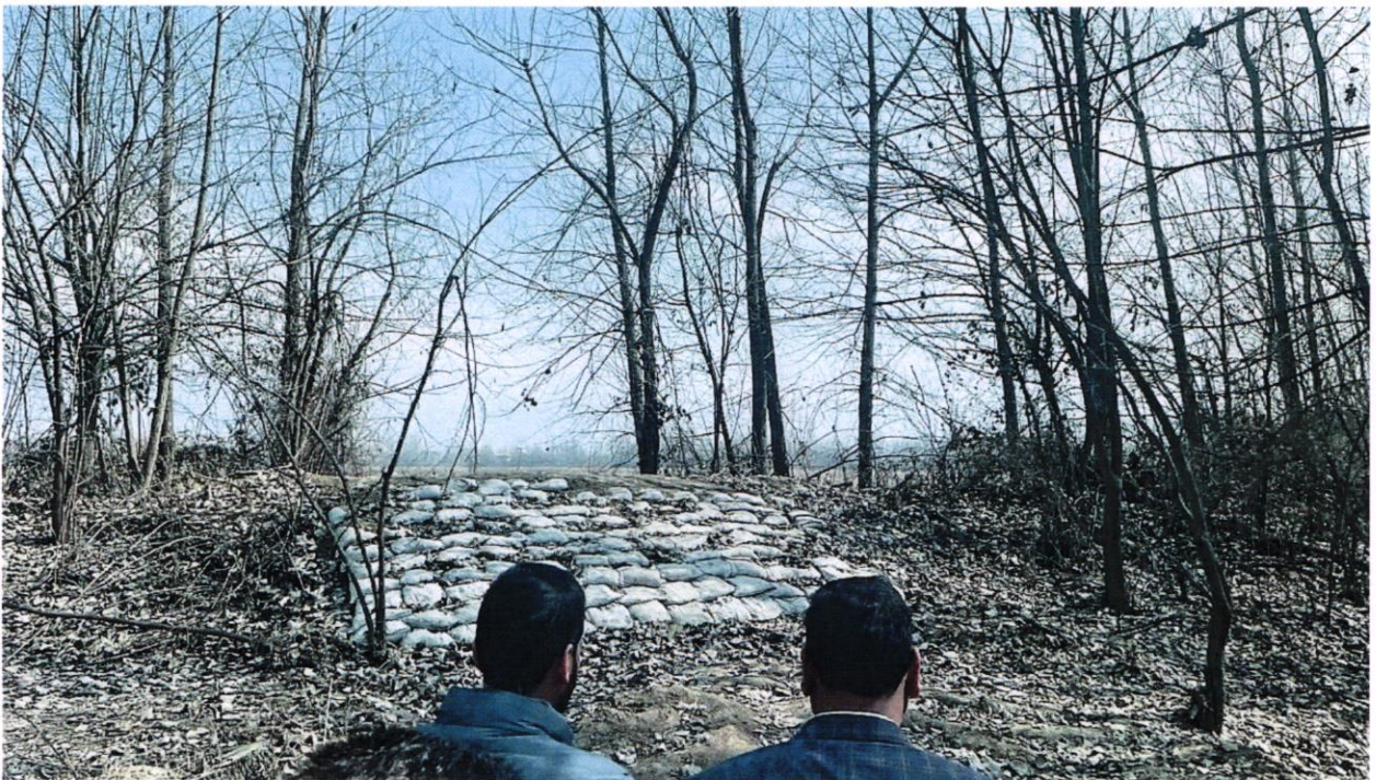
Photo 2. Embankment repaired by the Irrigation and Flood control department.
